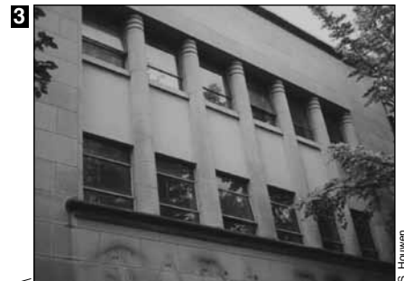
622 Granville, Saba Bros. Moderne facade at the Crewes Block
