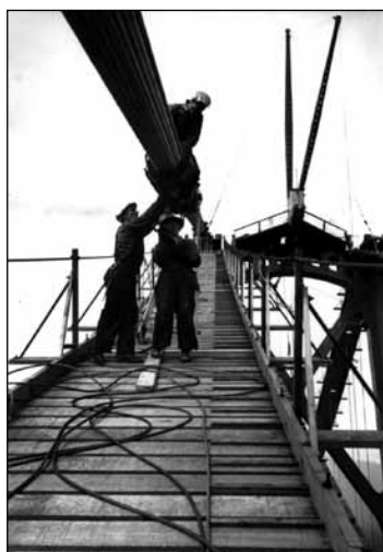
Construction of Lions Gate Bridge
