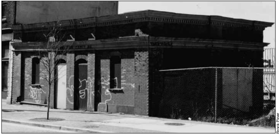
Gastown's CPR Telegraph Building the day before it was torn down late April.
